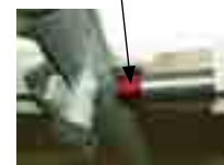
STOP SHOWN WHEN DOOR IS FULLY OPENED
